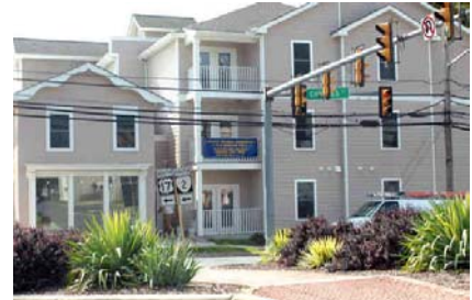
The Colonial Heights Apartments at Charles and Dixon streets in Fredericksburg are a blend of old and new. DAVE ELLIS/THE FREE LANCE-STAR
